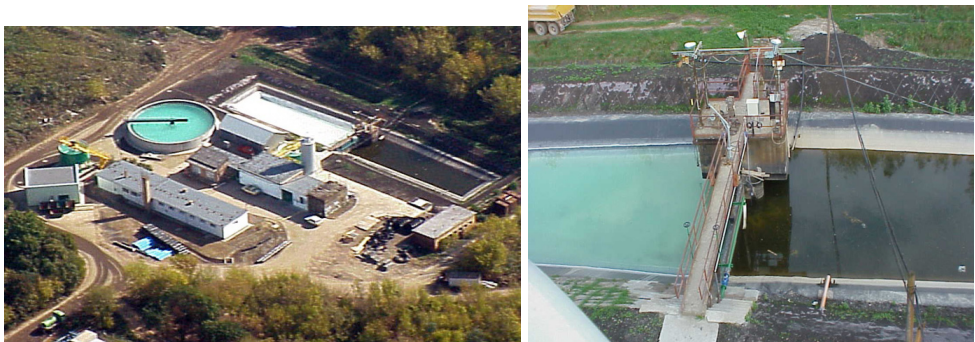
Fig.6 Wastewater treatment unit Mecsek (Pecs, Hungary) – general view, post-precipitation basin
