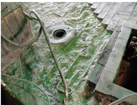
Figure 6. The appearance of the floor and fittings in the electrolysis plant
