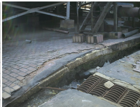
Figure 4. Raising the concrete foundation
