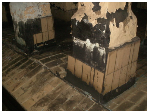
Figure 5. Supporting pillar electrolysis plant
