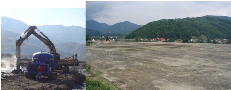
Fig. 10 Tailing pond remediation in Mojkovac, Montenegro: Deep mixing with mobile machinery, general view of the treated site
