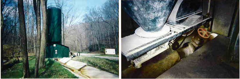
Fig.7 Acid mine drainage unit Snow Fork: General view, lime dosing powered by a water wheel
